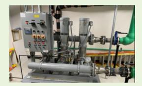
Existing System: (3) 20-horsepower singlespeed booster pumps
